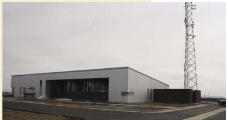
Above: Photo of the progress on the facility as of November 2009
